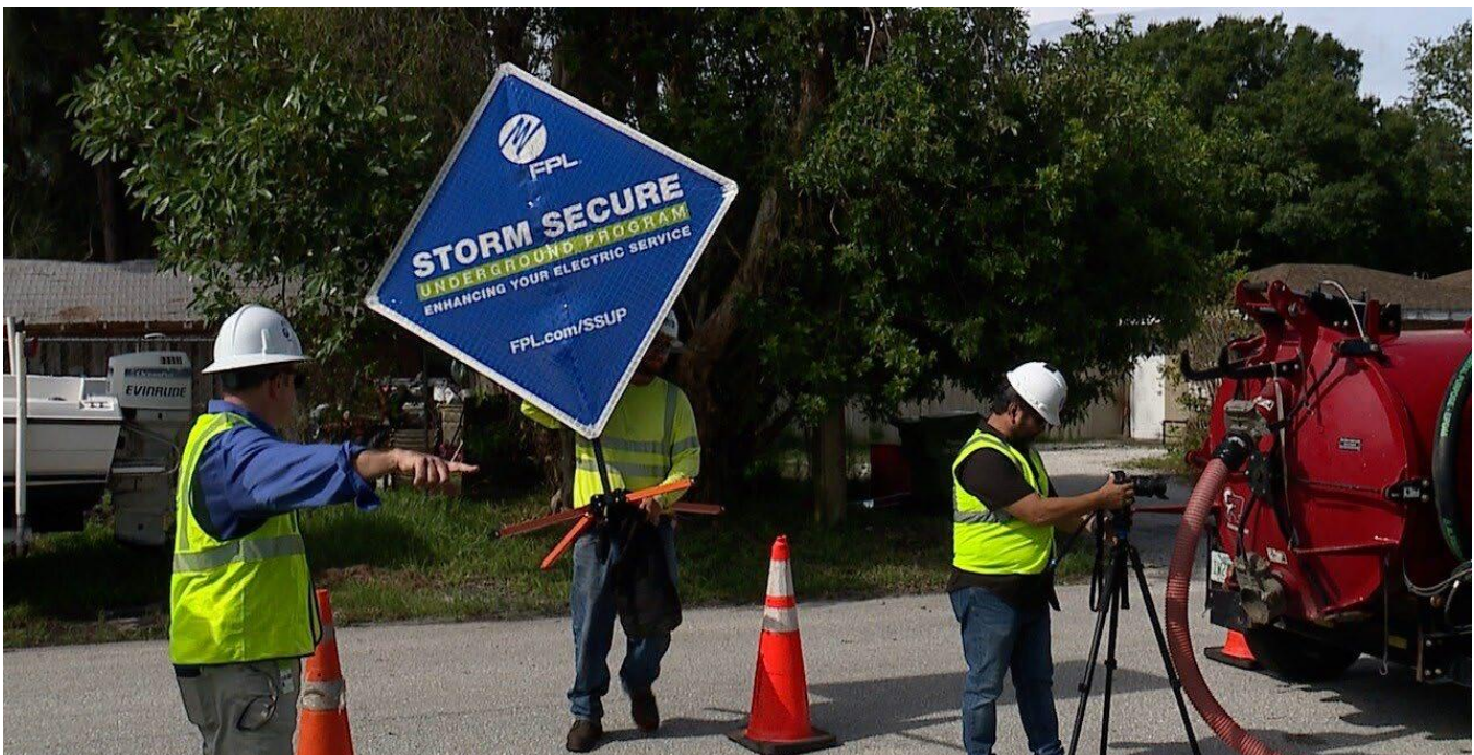
Photo: FPL Installing More Underground Power Lines
