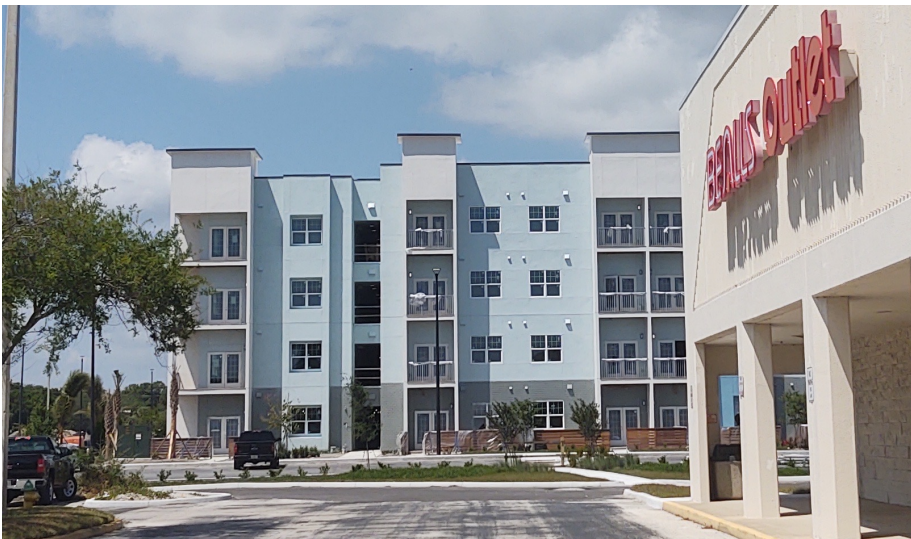
Image: Rockledge Flats, a 4-story residential project being constructed on part of a former Bealls anchored shopping plaza in Rockledge, FL.
